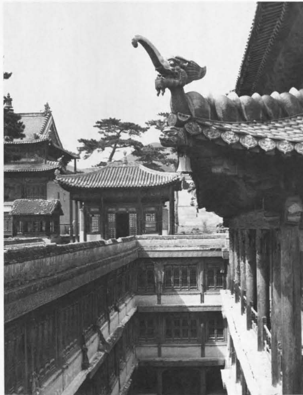
Roof of a pavilion within Hsü Mi Fu Shou Chih Miao.
