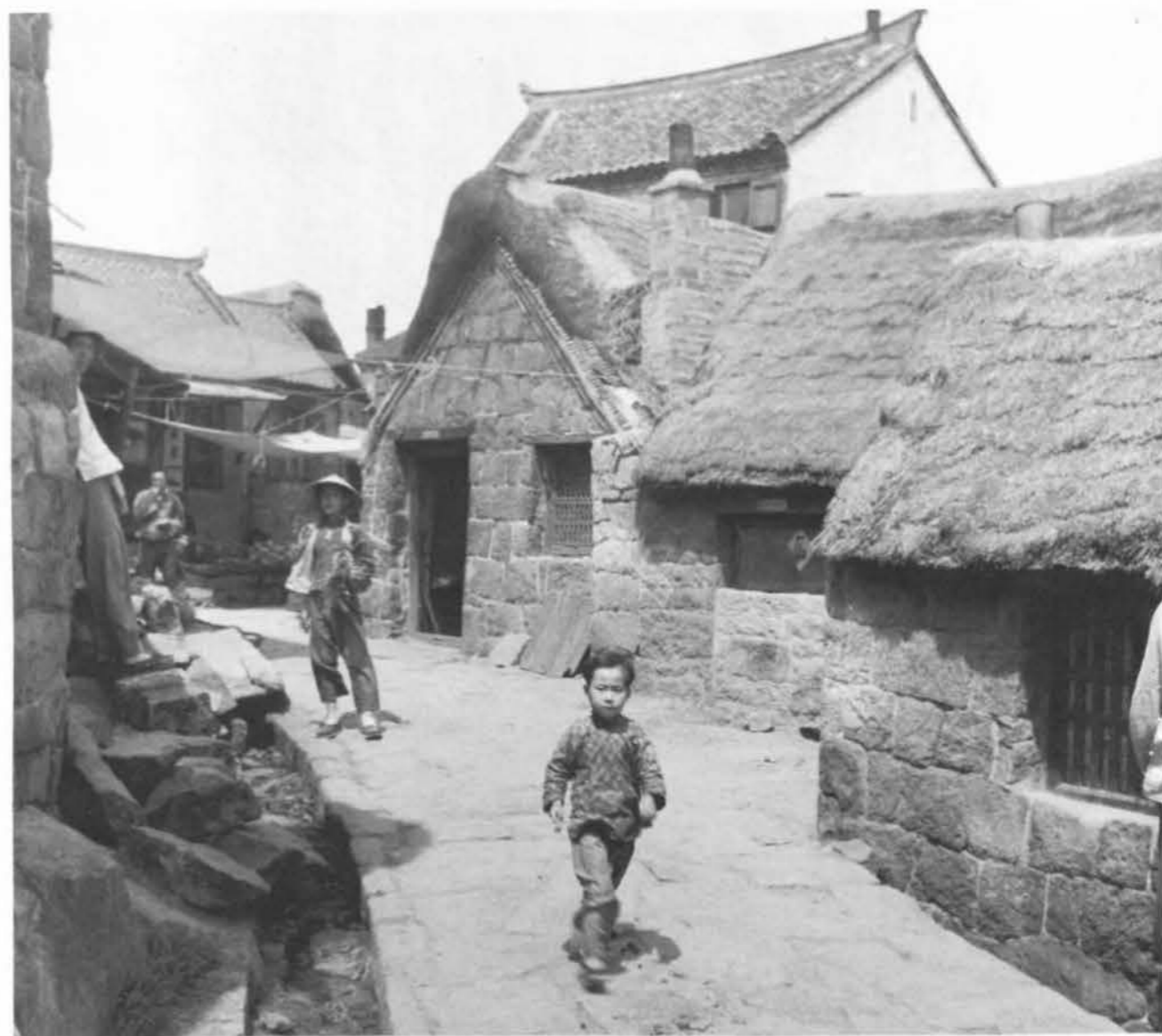
Even the poorer houses had massive stone walls.
