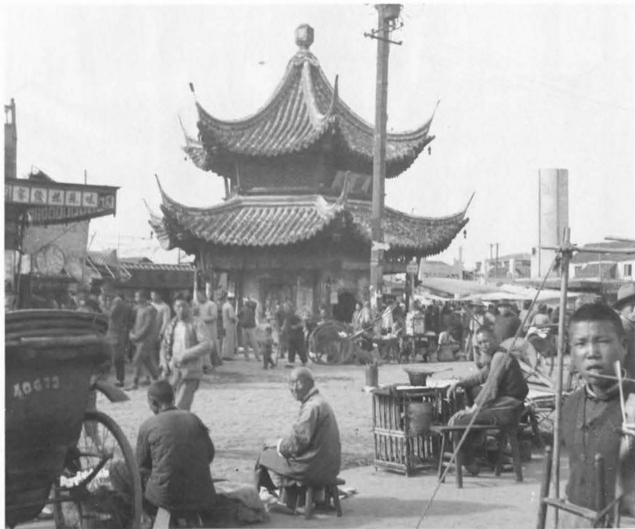
The Bell Pavilion housing the great bell which was the complement of the drum in the Drum Tower. The Pavilion is not the original building.
